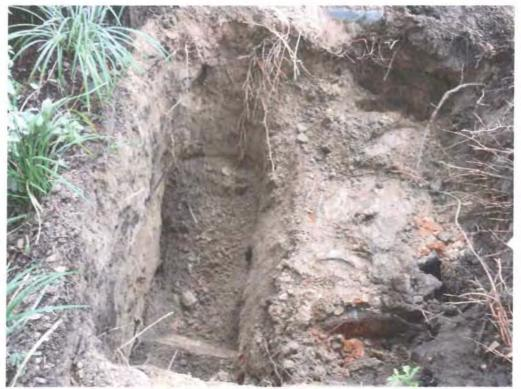
Picture 3: UST 159Cypress-2 excavation in progress.
